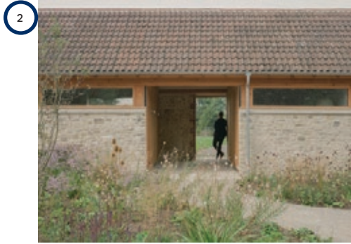
Fig 39. (2) Landscaping and Rainwater management system is key to bedding the Listed Barn back into its setting
