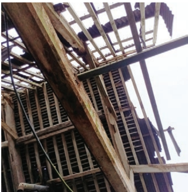
Fig 25. Existing Roof, March 2025
