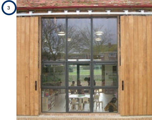
Fig 40. (3) Sympathetic Glazed windows and doors.
