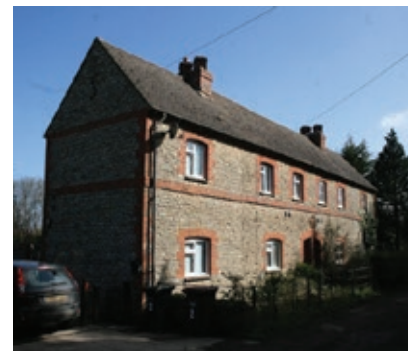
Fig 67. Buildings 16 and 17: Ashgrove Cottages, March 2022
