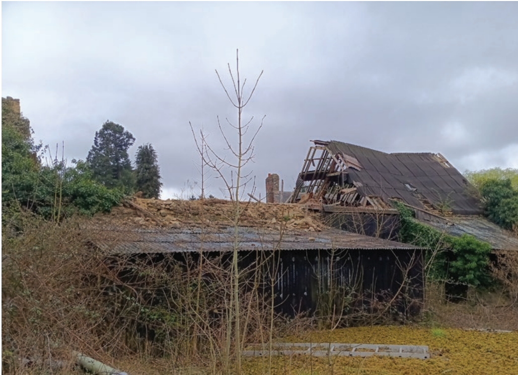
Fig 15. North elevation of Listed Barn building March 2025
