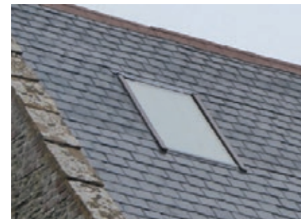
Fig 52. Rooflights to provide light to the space
