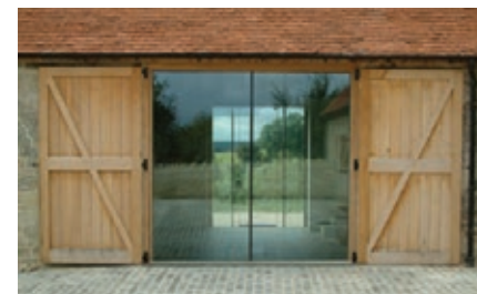
Fig 53. Entrance Barn Doors to signify entrance when open but be able to be perceived as shut with large barn doors
