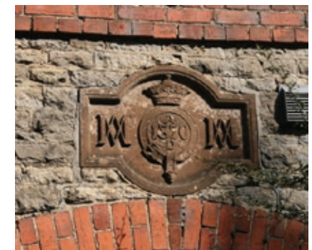
Fig 68. Buildings 16 and 17: Ashgrove Cottages, March 2022
