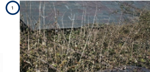
Fig 33. (1) Overgrown planting to be removed
