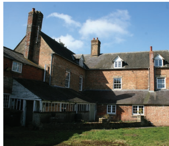
Fig 62. Building 9: Ashgrove Farm House, Rear Elevations, March 2022
