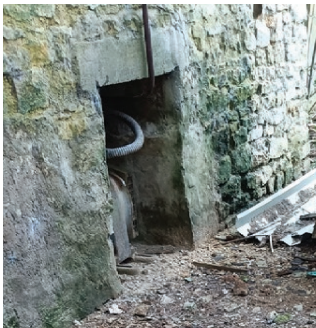
Fig 26. Existing Wall Bases, March 2025
