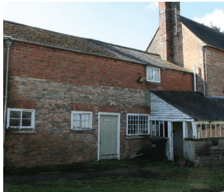
Fig 63. Building 11: Farmhouse Link, North Elevation, March 2022.
