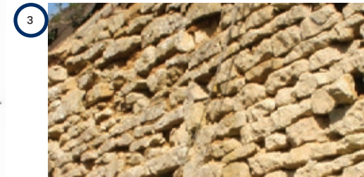
Fig 35. (3) Repair work and repainting to existing limestone walls
