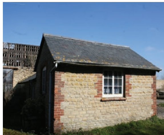
Fig 60. Building 3: Boiler Room, March 2022
