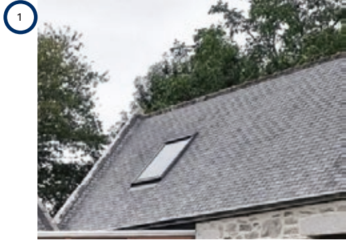
Fig 38. (1) Repaired Roof (see following review of design options)
