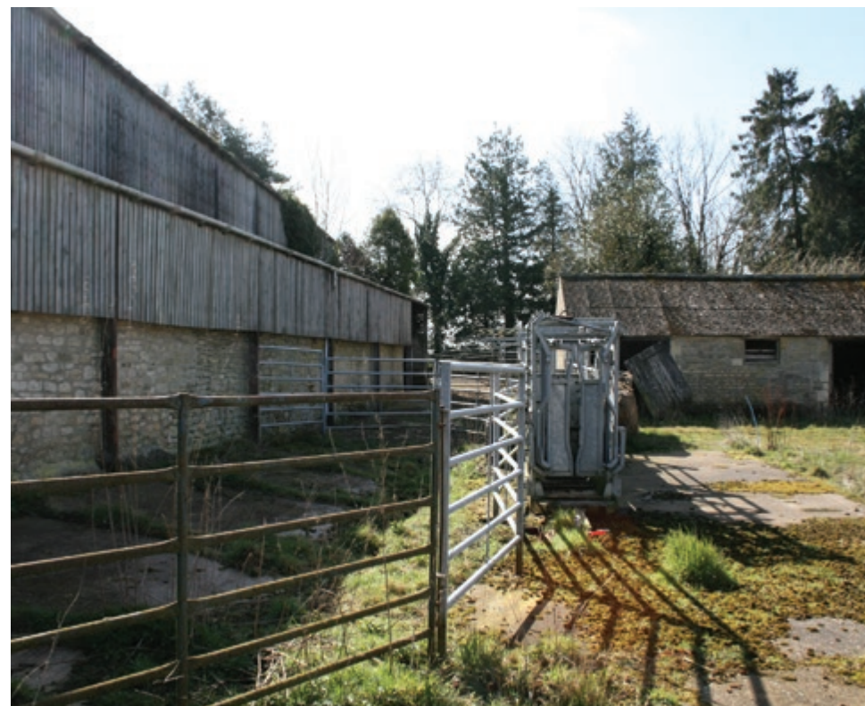
Fig 57. Modern Barn 19 sits partially on top of a historic wall 16 (due for retention). This may be suitable for dry storage of materials, or other equipment storage, during construction.
