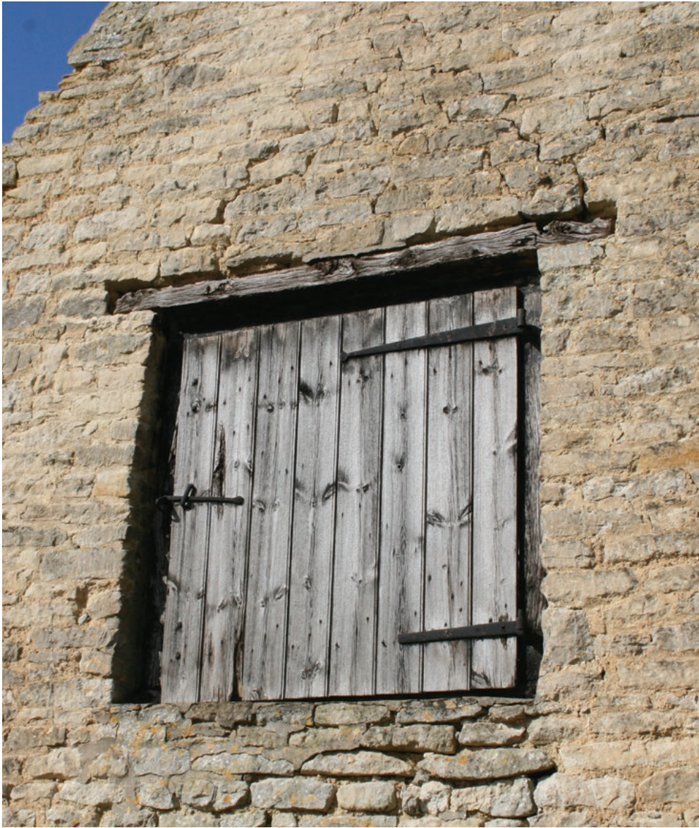
Fig 2. Listed Barn, East Gable, March 2022
