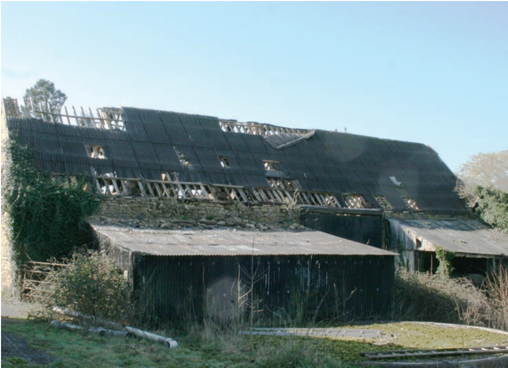
Fig 14. North elevation of Listed Barn building March 2022
